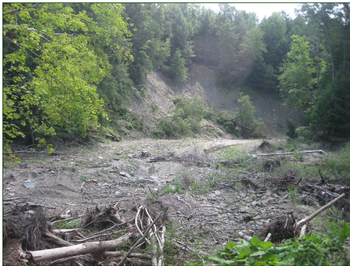
Figure 1: Banks of Wappasening Creek after Tropical Storm Lee
